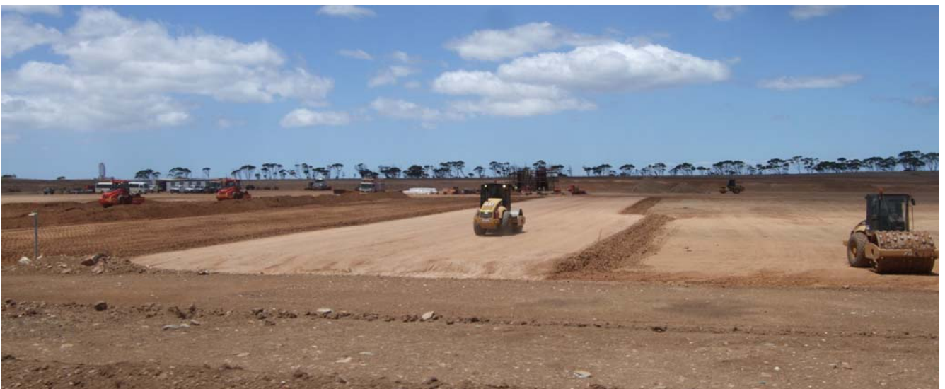
Bulk Earthworks progressing well
