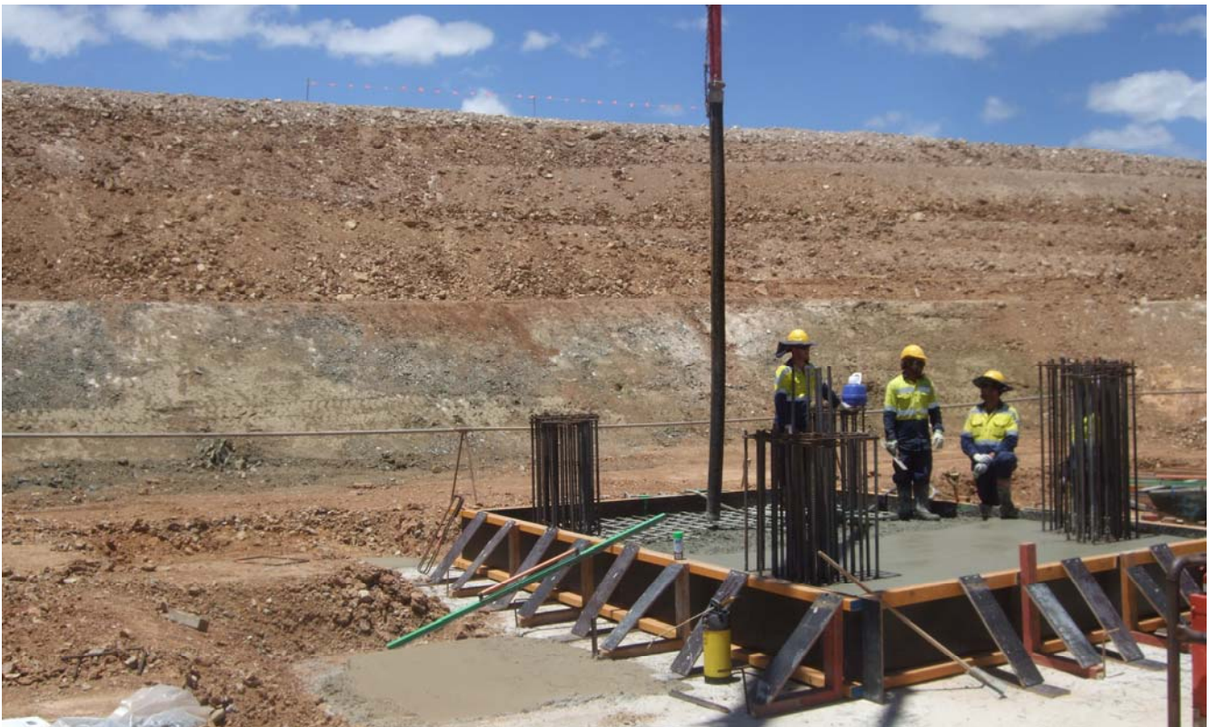
Run of Mine wall in the background
