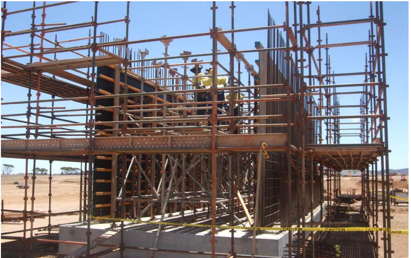
Fine Ore Bin form work ready for concrete pour
