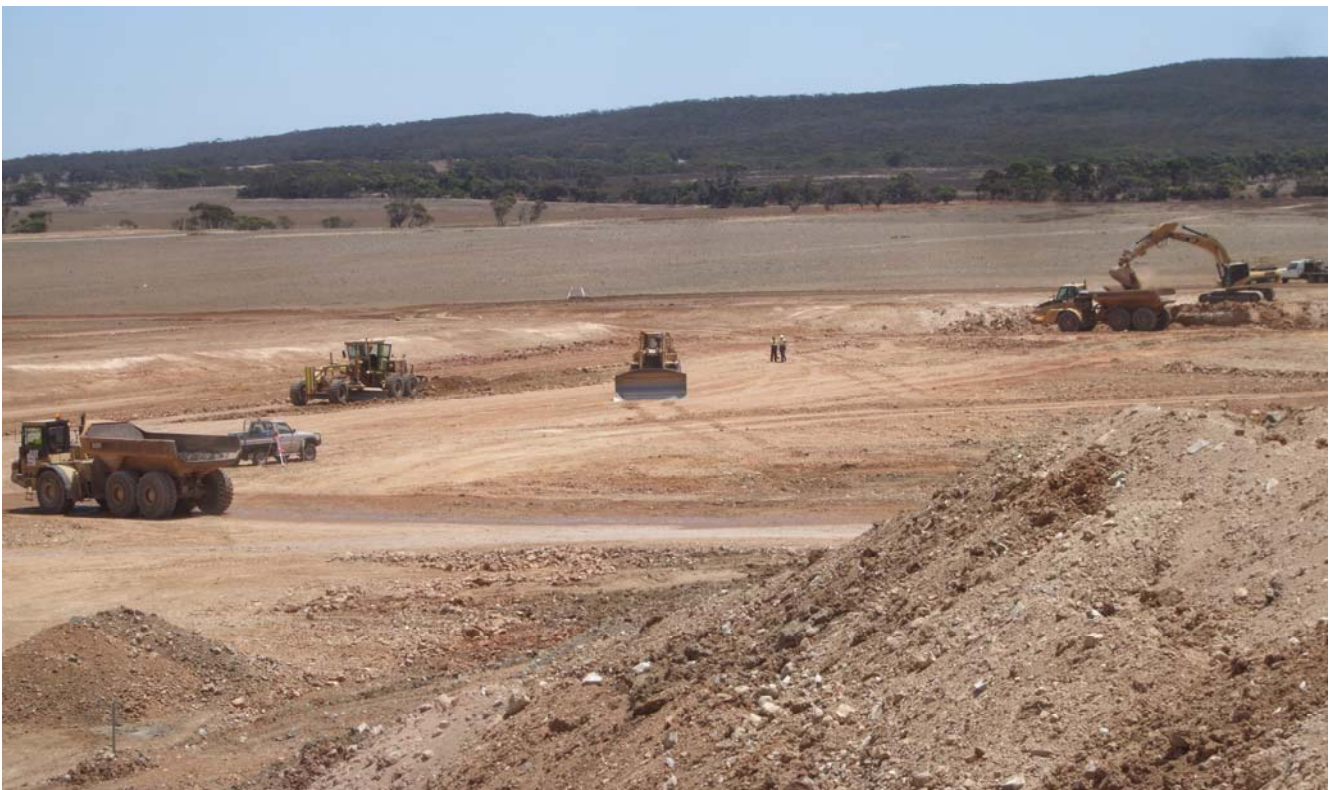
Bulk Earthworks from ROM pad
