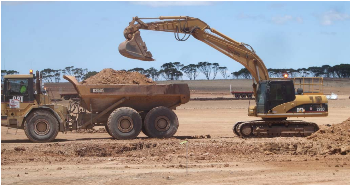
Excavator and Digger working on road access to Lake King Road
