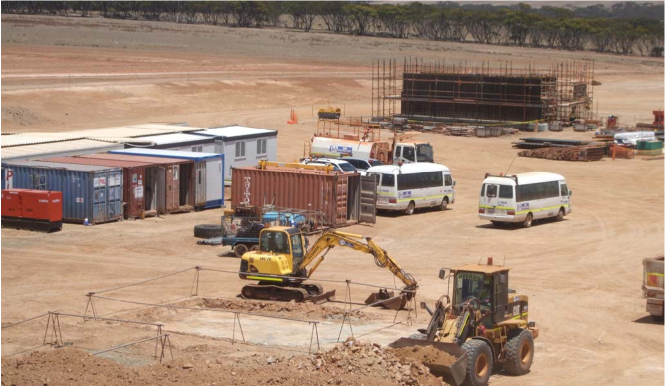
Fine Ore Bin concrete tunnel in background
