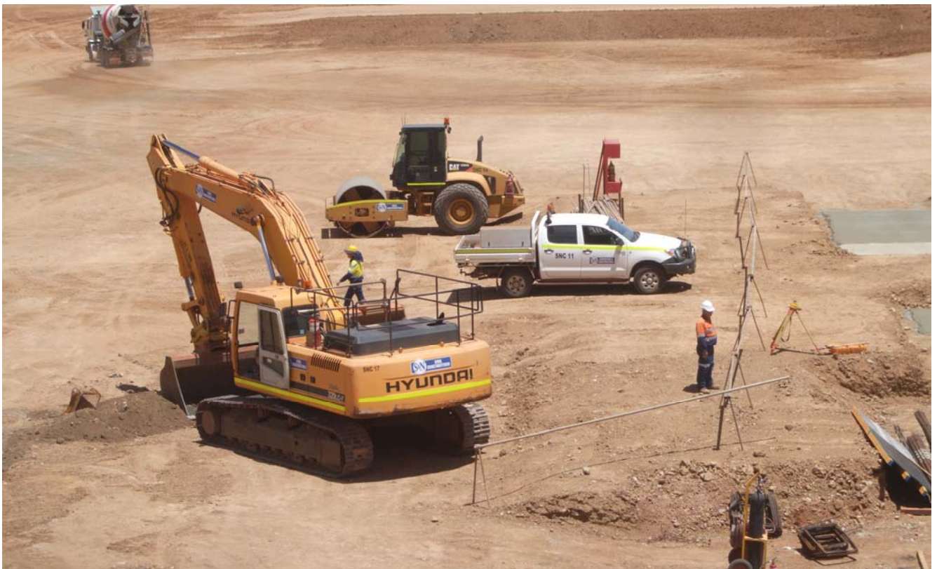
Bulk Earthworks expected to be completed by end Jan 2010
